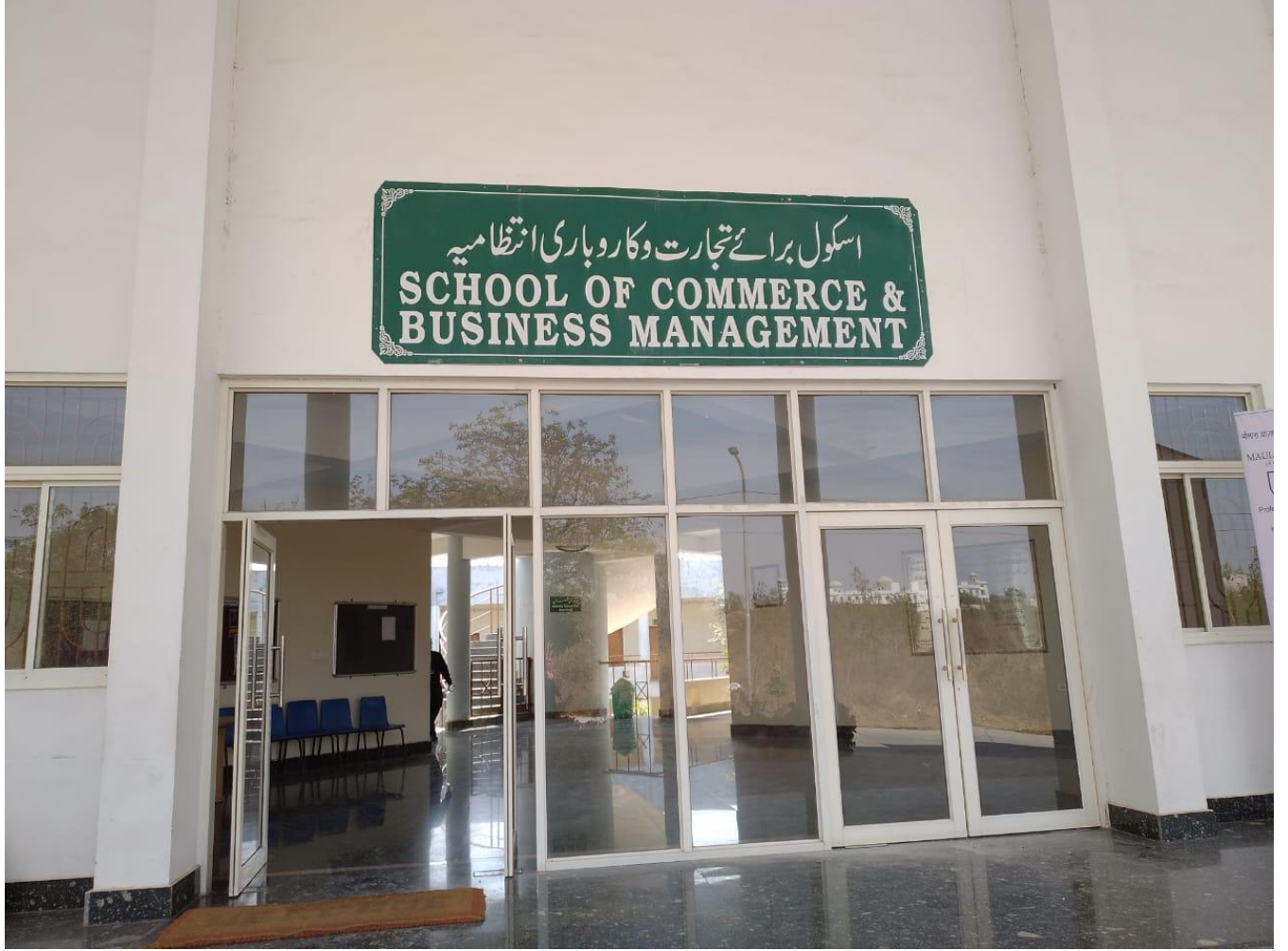
Entrance of the School building
